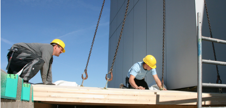
Assembly of a BBS flat roof element
