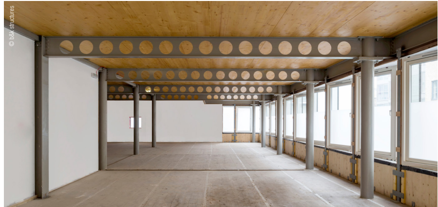
BBS elements resting on a steel structure
