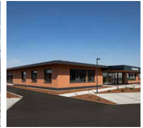
binderholz office building in Baruth | Germany
