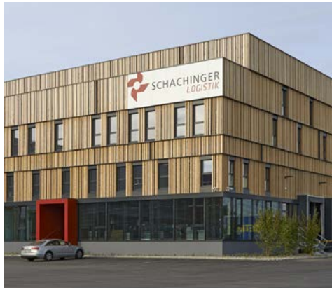
Logistikkhall Schachinger, Linz | A
