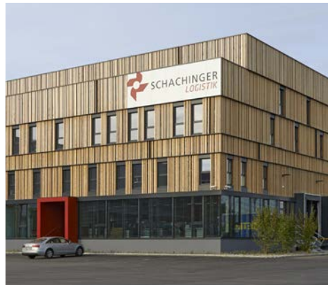
Logistikhalle Schachinger, Linz | A
